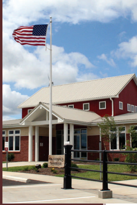
Metal roofs reduce heat island effect
