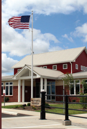
Metal roofs reduce heat island effect
